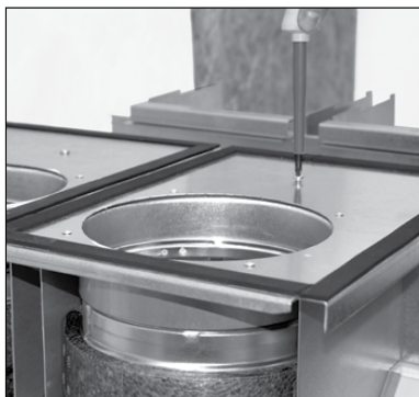
8. Secure two end piece plates with one screw each
