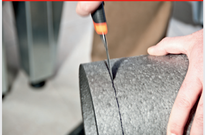
Cutting ComfoPipe to Length
