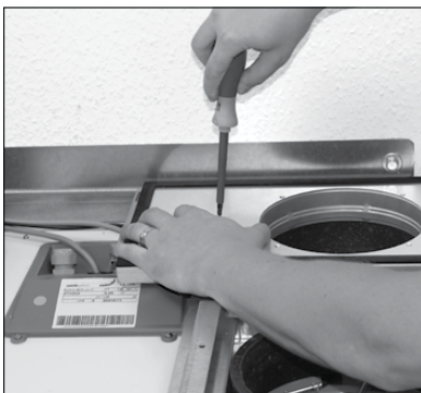
7. Secure end piece plate with one screw
