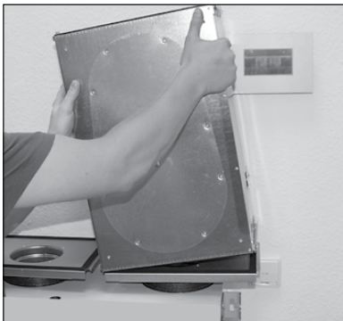
4. Place attenuator on the end plate
