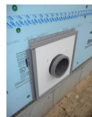
Mounting block installed over Roflex gasket
