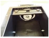
Keep spare disks and installation manual in a plastic bag close to ComfoAir Ventilation device for further adjustments.
