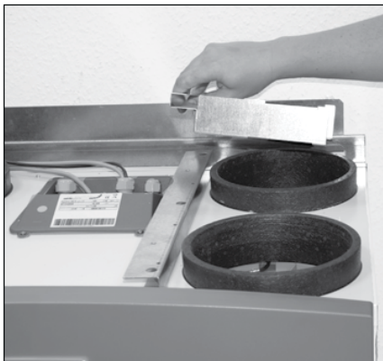
4. Attach the mountings to the U-profile
