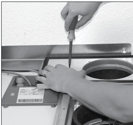
7. Secure end piece plate with one screw
